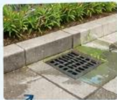
Regard, avaloir, évacuation...
